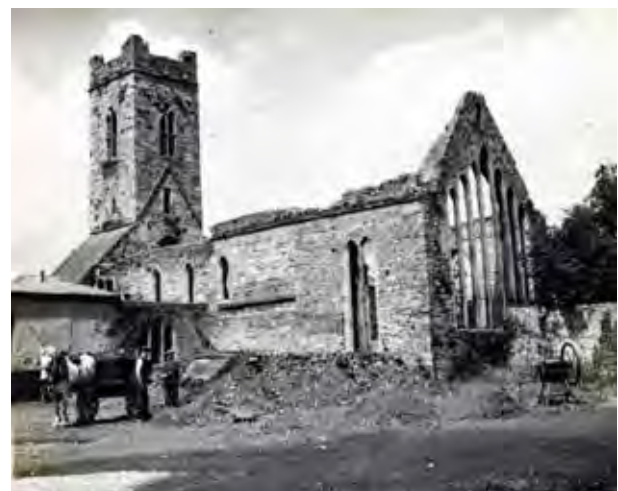
Fig 42. 1946, the Abbey following restoration works, horizontal bars are still visible supporting the east window.
