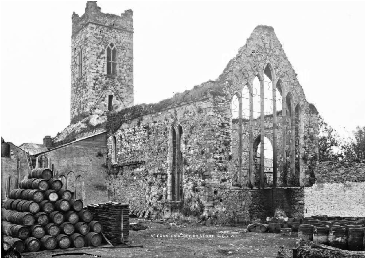
Fig 49. A view of the east window in the 1880's when the building was used as part of the brewery. Notice the iron rods supporting the mullions
