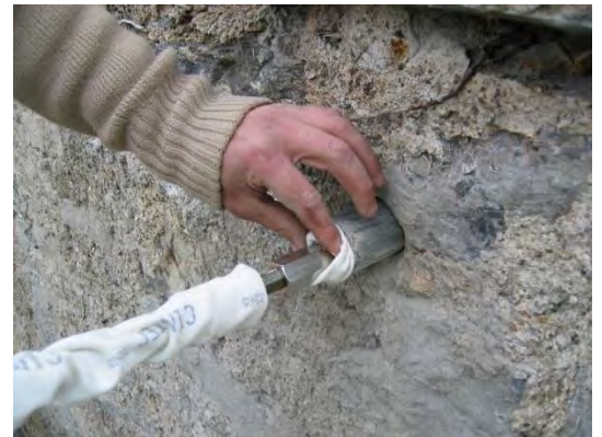
Cintec anchor installation to a barbican tower. These ties extended up to 9m thro the tower. The outer metal sleeve that forms part of the coring procedure is withdrawn before grouting.
