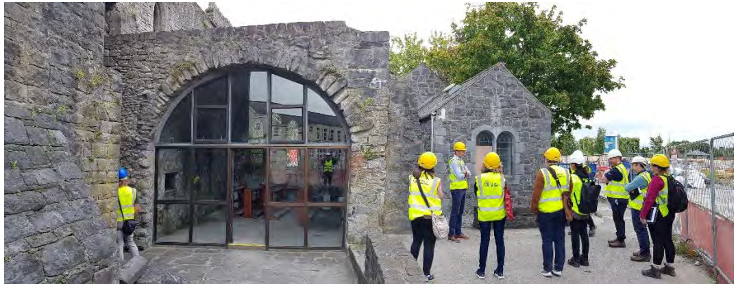
Sacristy – note little overburden to arch and lean of right-hand side supporting wall.
