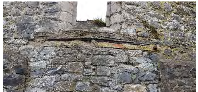
Steel lintel to previous doorway west end of north wall
