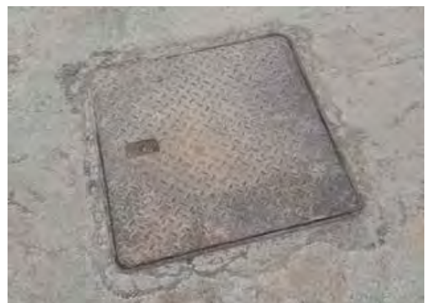
Fig 50. The only evidence of the well, the manhole leading down into the concrete chamber below.
