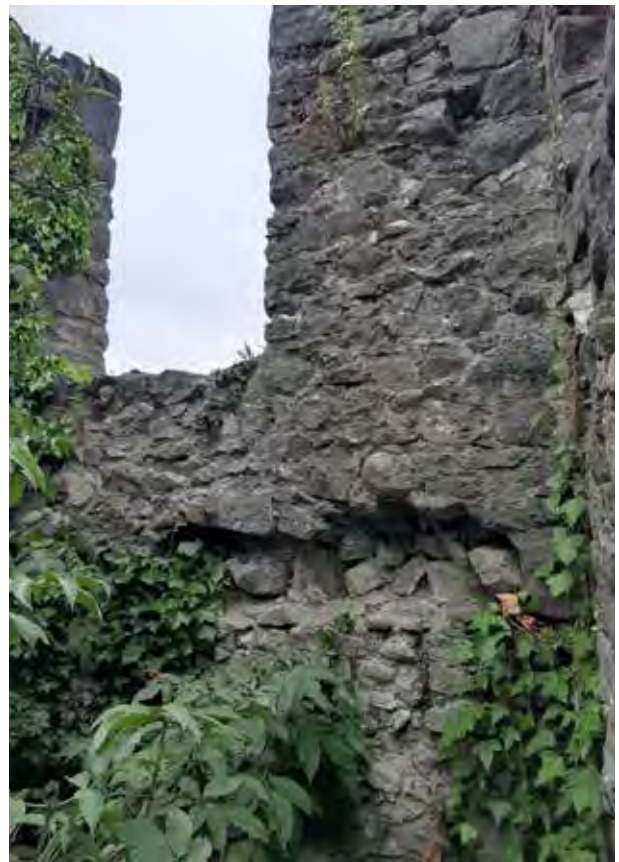
Fig 68. Interior of the turret showing locations where floor timbers may originally have been
