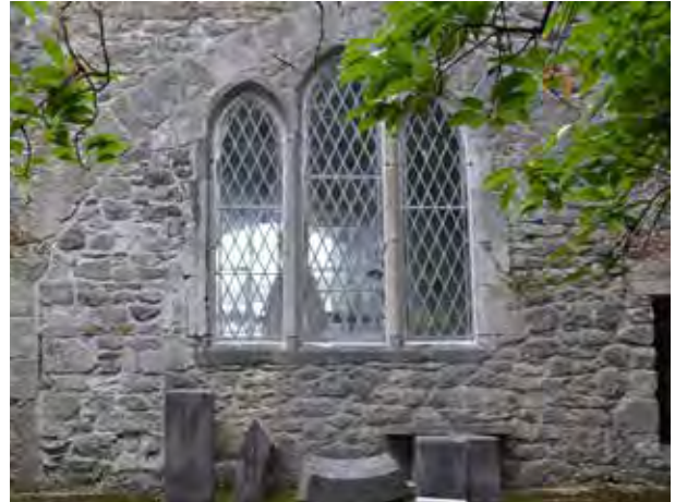
Fig 82. External view of the sacristy east wall , showing the infilled arch and window
