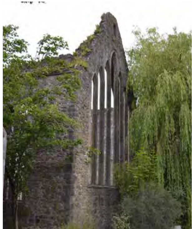
Fig 96. The east window showing the large willow tree encroaching on it.
