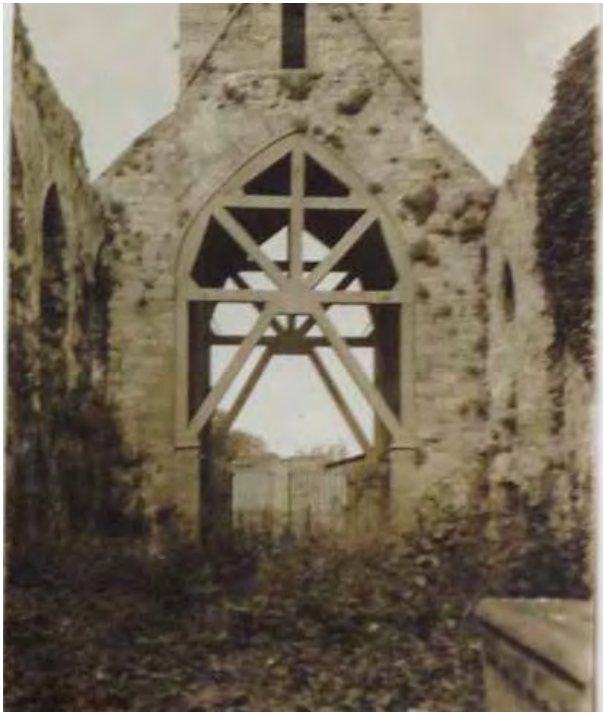
Fig 33. 1926, original timber formwork to the Abbey (Courtesy of the Photographic Archive, National Monuments Service)
