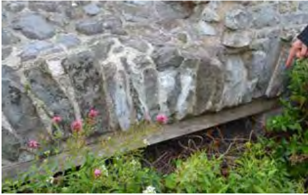
Fig 62. New timber supporting relieving arch in city wall
