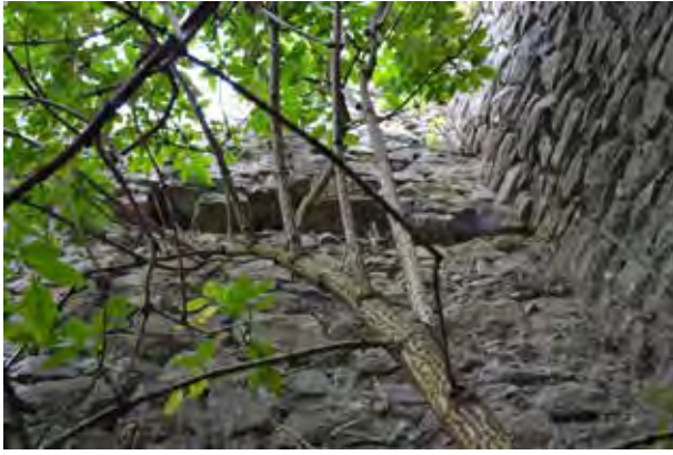
Fig 66. Large tree growing in the interior of Evan's Turret
