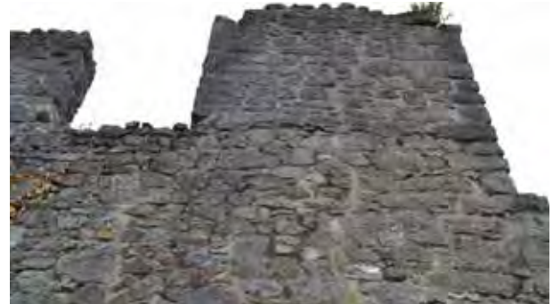
Fig 64. Detail of the facade of Evan's turret showing the different layers of construction
