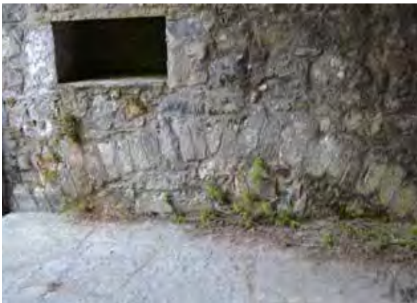
Fig 81. Relieving arch in north wall of the sacristy
