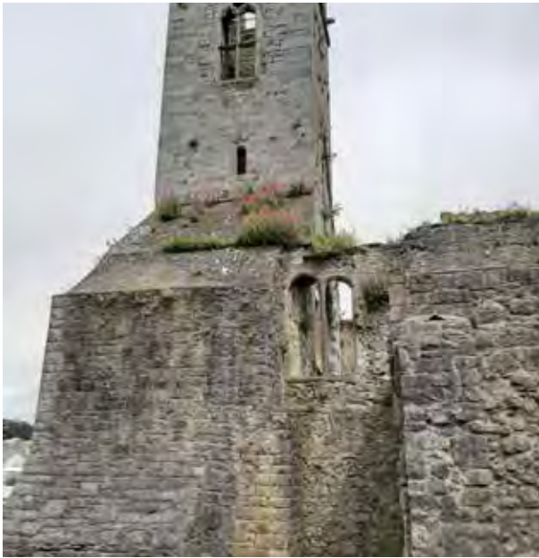
Fig 74. Newer buttress to the south of the tower
