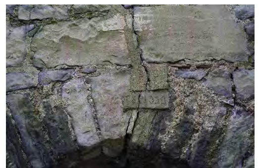
Detail of 1949 and 1987 cement mortar tell tails. Photo c/o Chris Corlet
