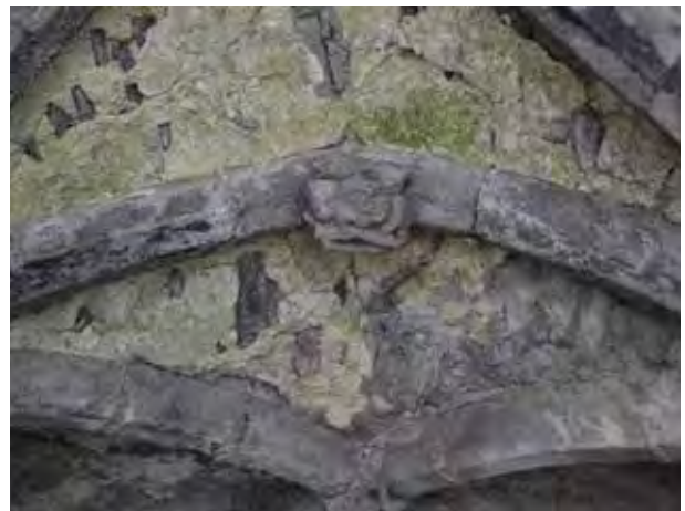
Fig 40. Rib vaulting to the underside of the passage from the tower
