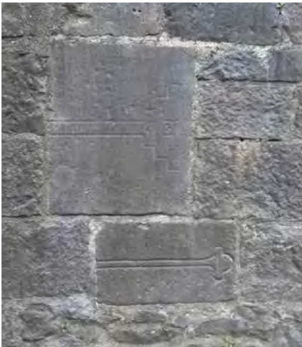
Fig 97. Grave-stones incorporated into the east wall below the large window.
