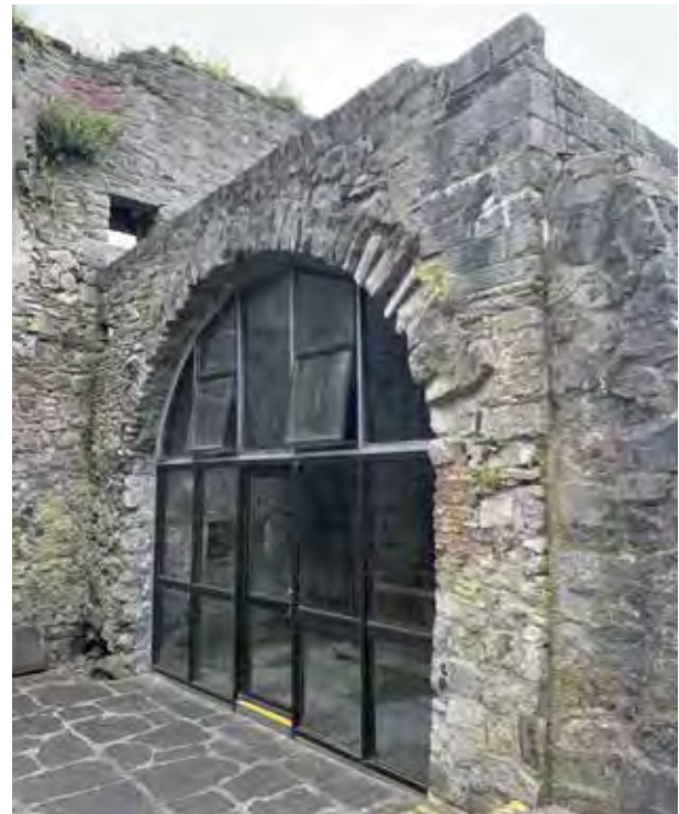
Fig 79. In-filled glazing system into the Sacristry'
