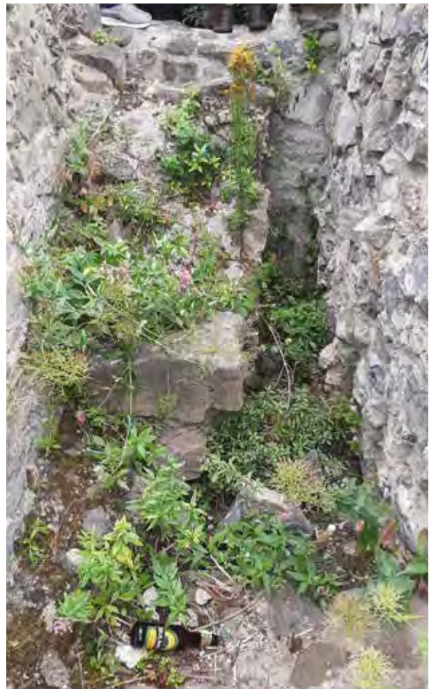
Fig 103. Vegetation growing on the wall walk within Evan's turret.
