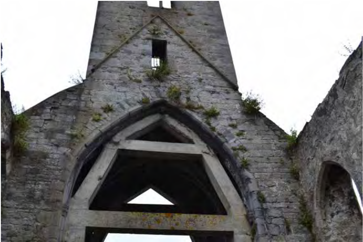
Fig 36. The concrete supports in-situ today
