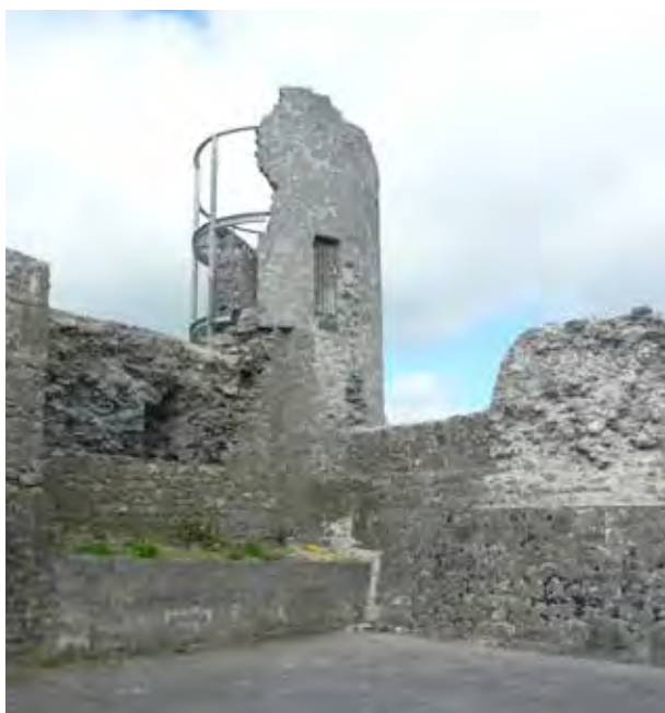
Fig 109. Stainless steel spiral stair inserted in the north west tower in Athenry (by HHC Architecture)
