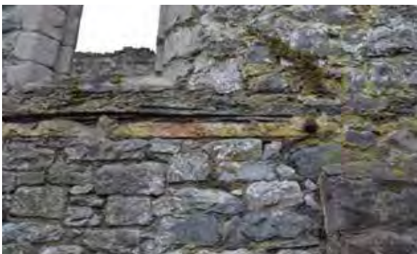
Fig 72. Corroded metal beam where a new opening was made in the wall
