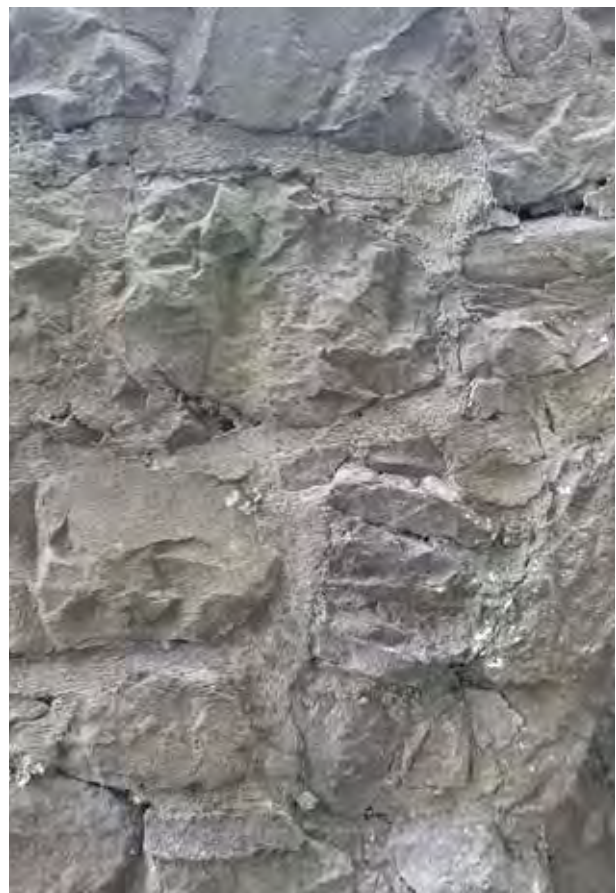
Fig 101. Stones poorly pointed with cement pointing in the east wall.
